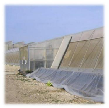
Protection of ventilation openings with insect nets
